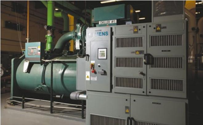
Figure 5: Siemens SINAMICS Perfect Harmony VFD installed at Mirage chiller plant
