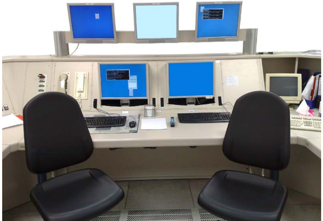
Figure 1. A fresh look. A new automation system provides power plant operators with a better view into the process via PC-based HMIs and should also include an improved alarm management regime.
