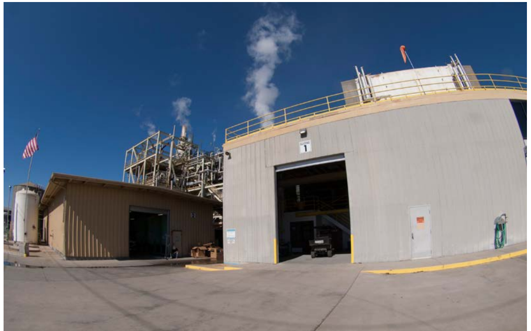
Figure 2. Upgrade time. The existing DCS at this cogeneration plant needed to be replaced to improve operations, cut downtime and minimize maintenance.
