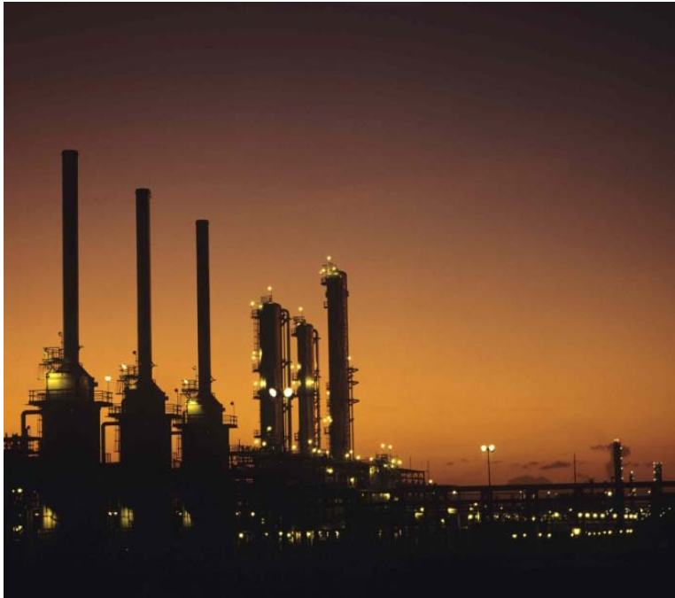
Figure 1. For certain industries, a DCS provide substantially more value as the basis for automating the plant than a PLC-based system.
