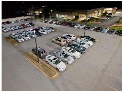
270 Watt LED fixtures producing 4 measurable foot candles
